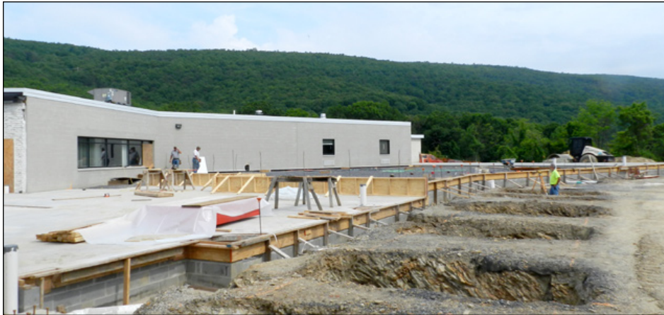
New Construction at Friends Aware
